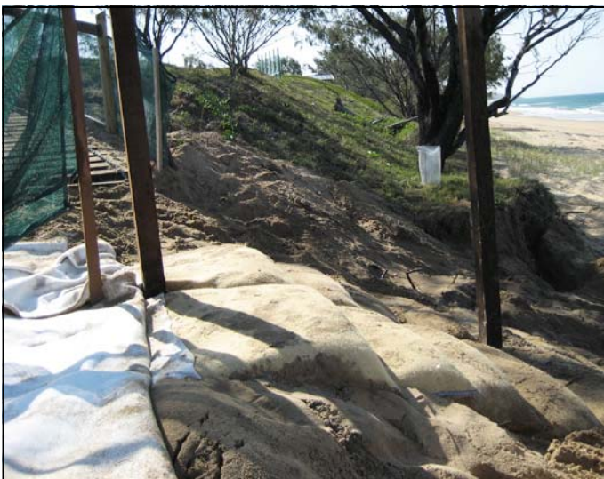
Construction almost complete
