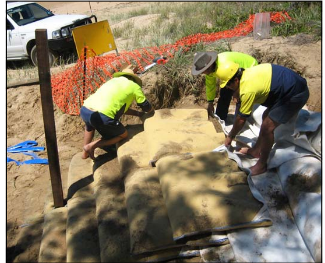
ELCOROCK® containers during construction
