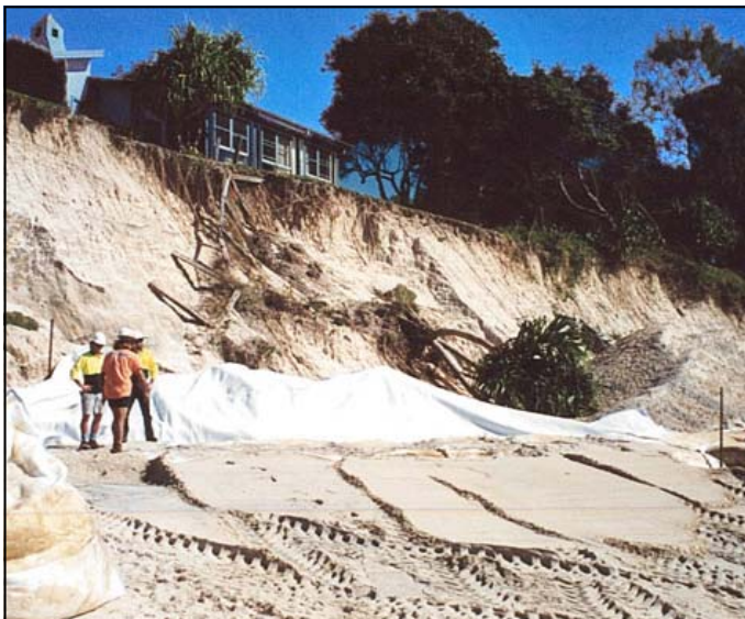
House in danger
