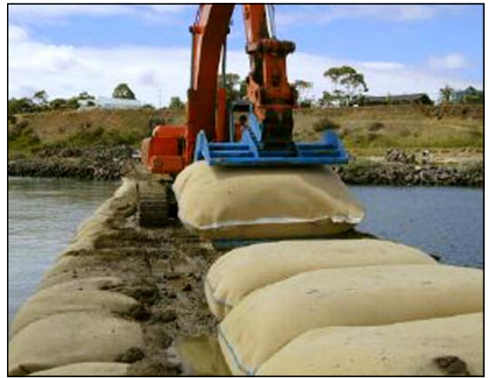
Placing the ELCOROCK® containers
