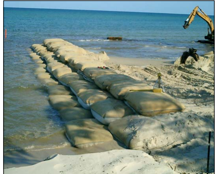
During construction of groynes
