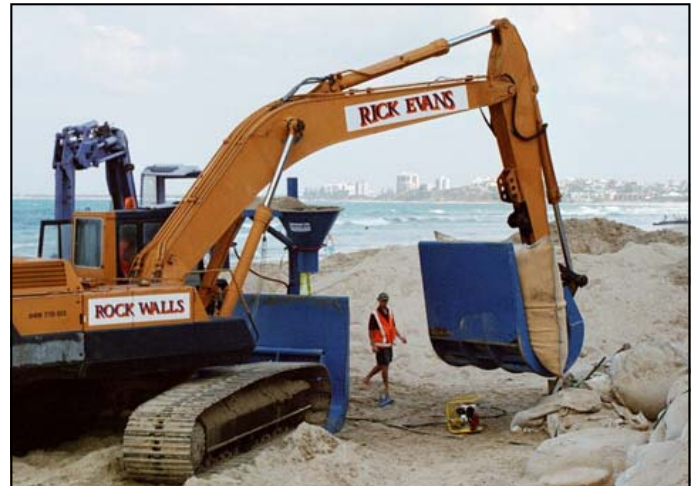
Filling and placement of the ELCOROCK® containers
