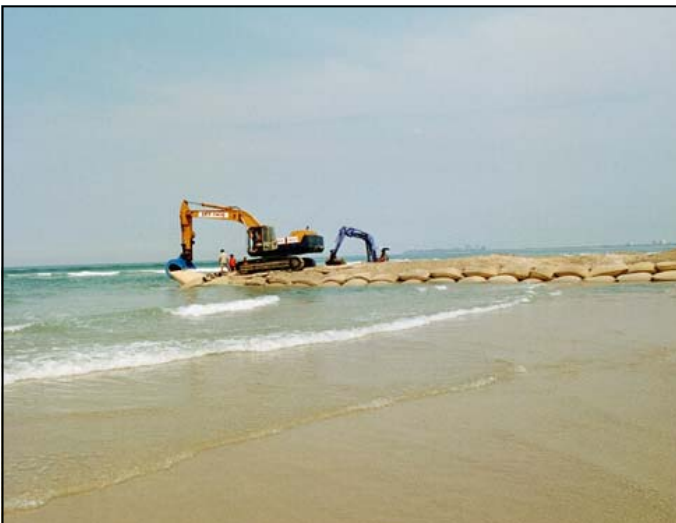
Placing the ELCOROCK® containers
