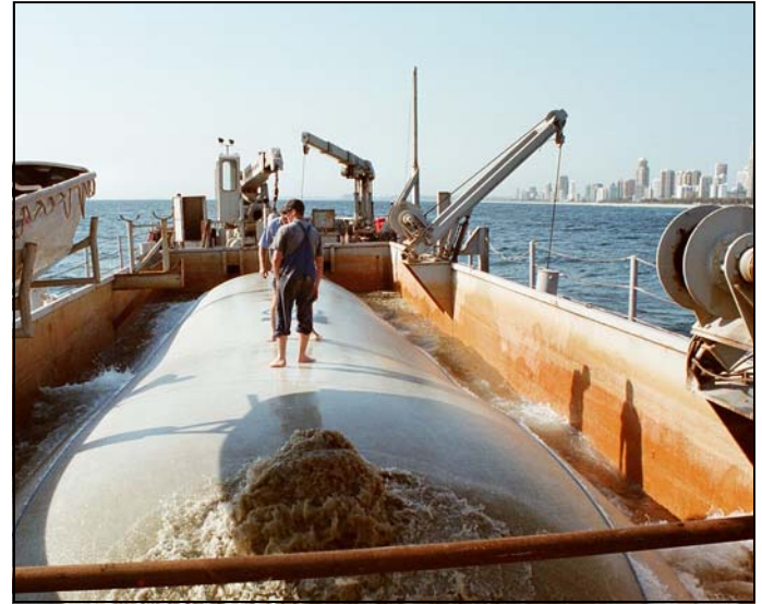
Placement of ELCOROCK® Mega Containers
