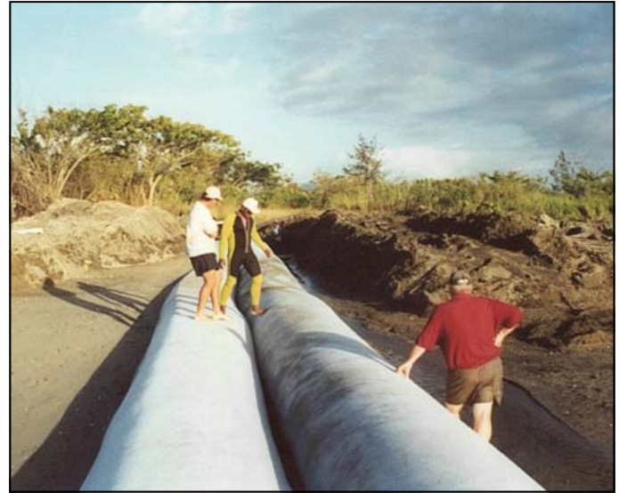
Installation of 2 base tubes
