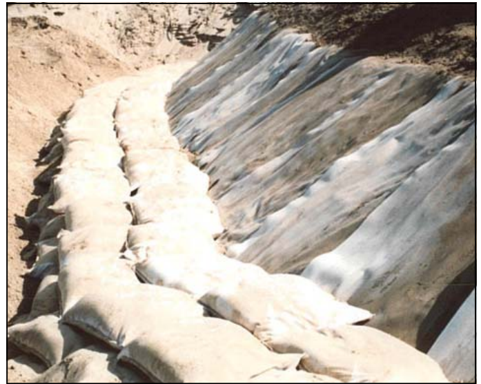
During construction – ELCOMAX® install under ELCOROCK®
